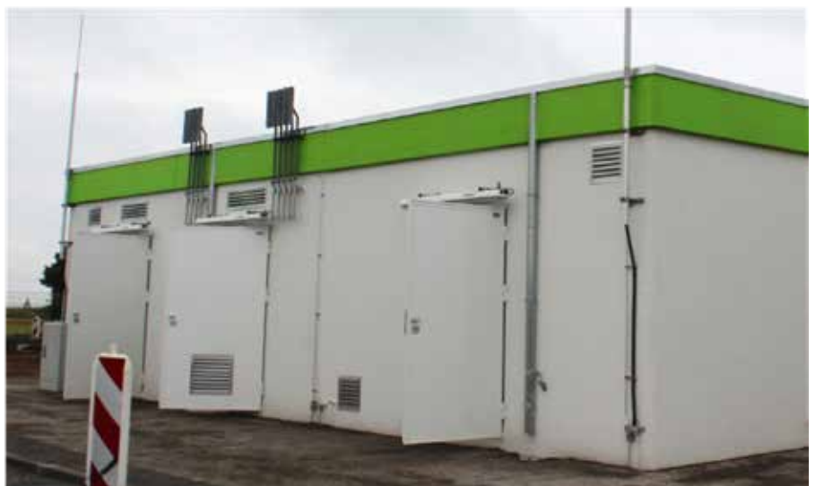
Abb. 7: Wall and pipe mounting: Internally routed isCon ® arrester in air-termination rod in biogas plant
